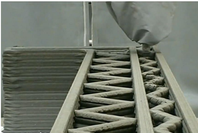
Fig. 2. Walls created in Contour Crafting technology [14]
