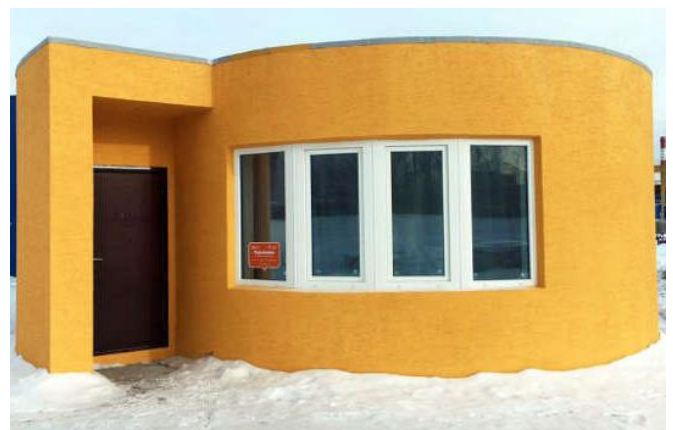
Fig. 5. House made according to the design of Apis Cor in 3D printing technology [13]
