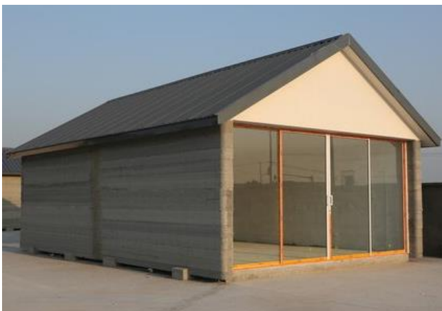
Fig. 3. Single-story building made by WinSun in 3D printing technology [20]
